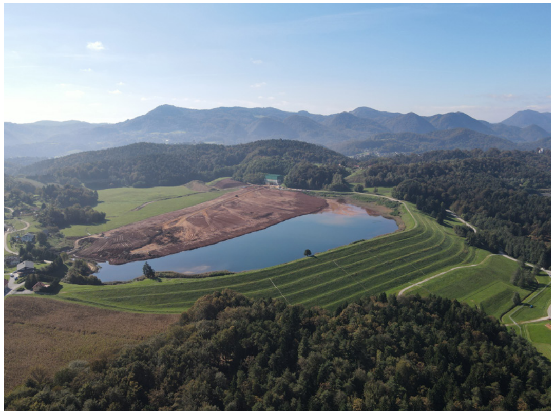
Za Travnik – a waste disposal facility
